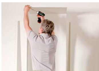
Screw front corner in place with a cordless screwdriver. This makes one-person assembly easy
