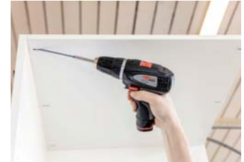
4. Connect the workpieces
