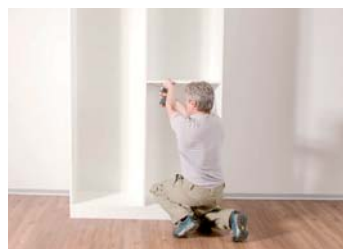
Tip: - Place one side of the shelf on the shelf support and fasten the other side - Screws loosened flush simplify installation
