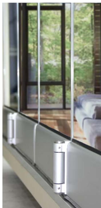
Weather proofing brush between bottom profile and the floor.
